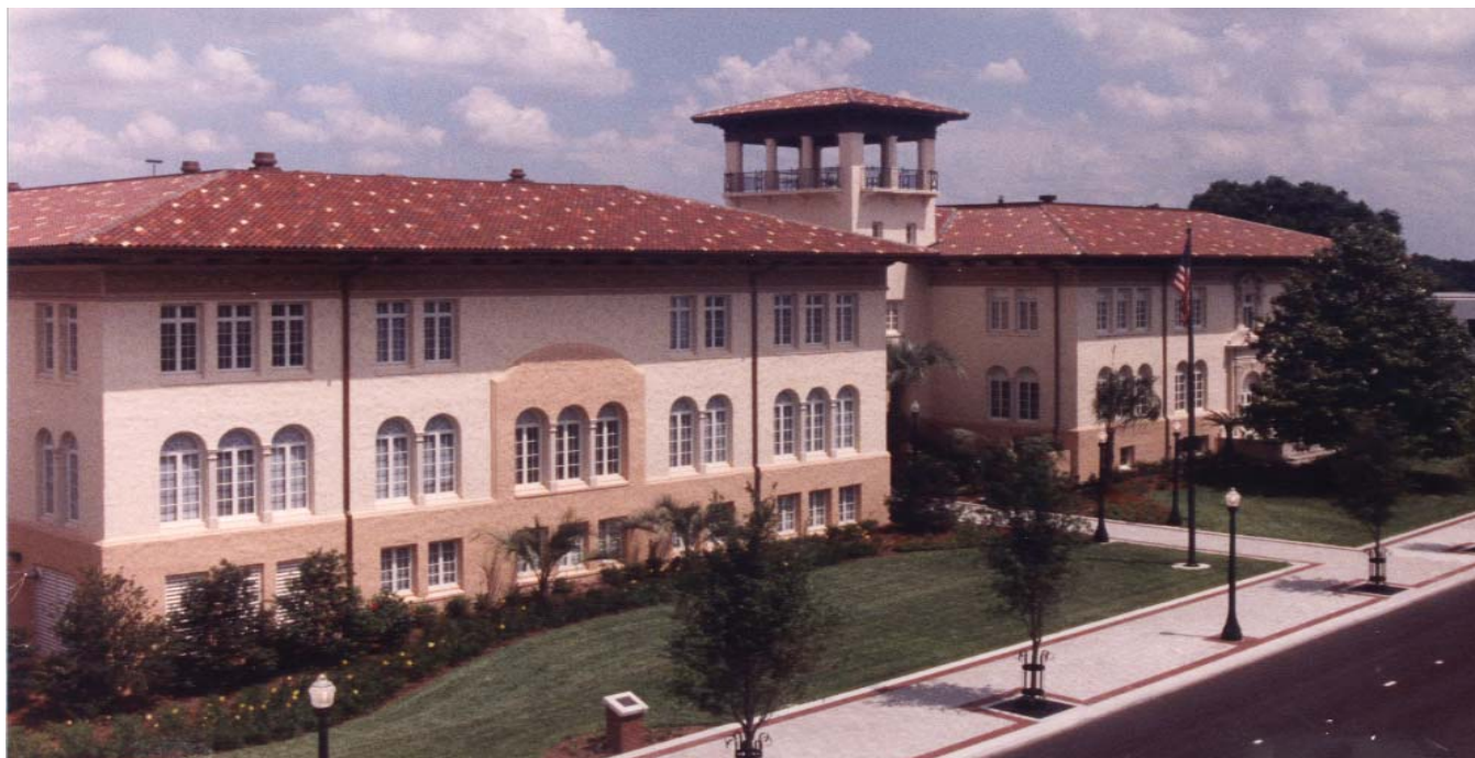
40,000 SF addition to City Hall which became a “fraternal” twin to the historic original and incorporates the City Commission Chamber
