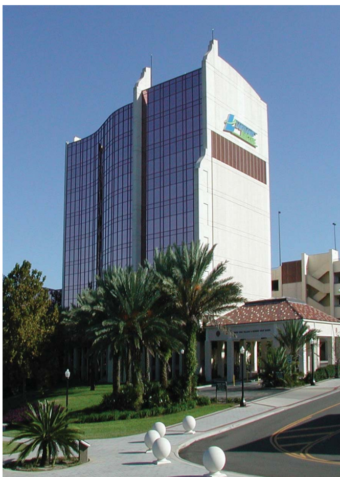
110,000 SF, ten-story administration center for Lakeland Electric & Water including a secure 24 hour operation center and a 518 car garage
